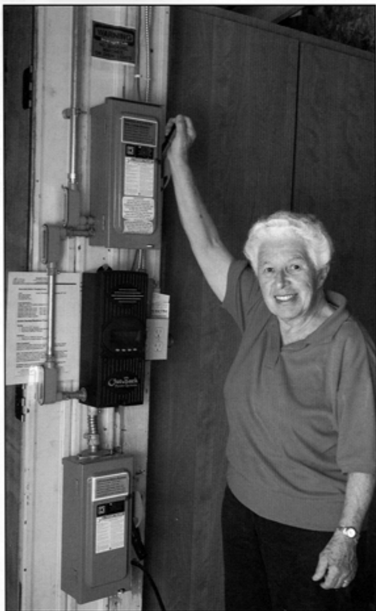
S. Paula Gonzalez showcases the operating system used to convert sunlight collected by solar panels on the roof of her home, La Casa del Sol, into energy, which charges the battery that powers her golf cart.
